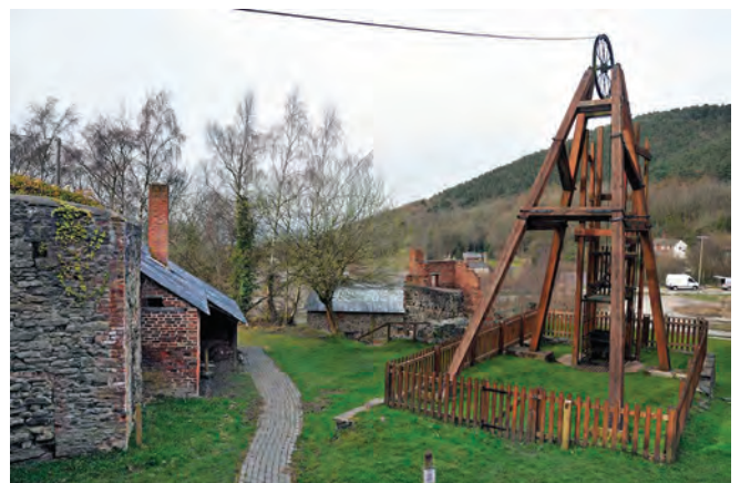
The reconstructed wooden headframe over the George's Shaft at Snailbeach
